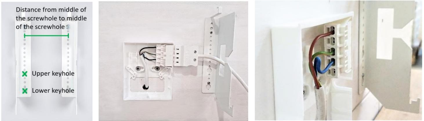
Note safety distances when mounting the heater on a wall. The safety distance is 50mm on each side and 100mm upwards. The recommended minimum height is 50mm off the floor. The thermostat adds 50mm to the width. The distance from the wall to the front surface of Walo heaters is 110mm and 75mm to the front surface of Warma and Wahva heaters, but 100mm to the thermostat's front surface.
